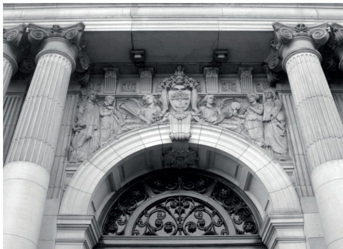
Fig. 4: City Chambers main entrance archway frieze, central panel. (Author's Photograph)
